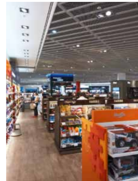
The conditioned air is blown draught-free via slotted rails into the retail areas.
