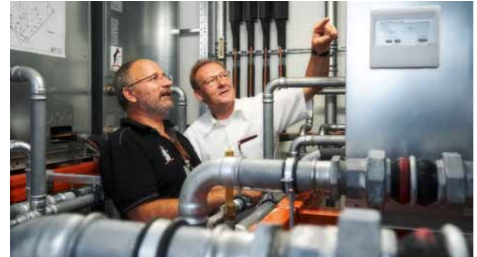
Rolf Wiesinger (W+W Kälte- und Klimaanlage GmbH) and Thomas Schmidt (Mitsubishi Electric Frankfurt) during the function testing of the first ready-to-use installation.
