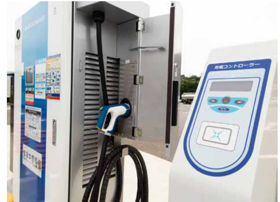
In Japan there are many more charging points than conventional petrol stations.
